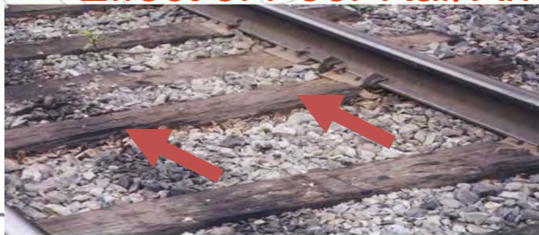
Effect of Poor Rail Anchoring
