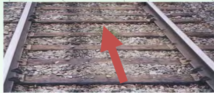
Effect of Poor Rail Anchoring
